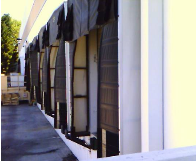
Figure 7 – Some Docks at Fremont Lean Logistics Center
